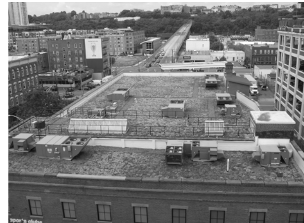
Green Roof in Hoboken
