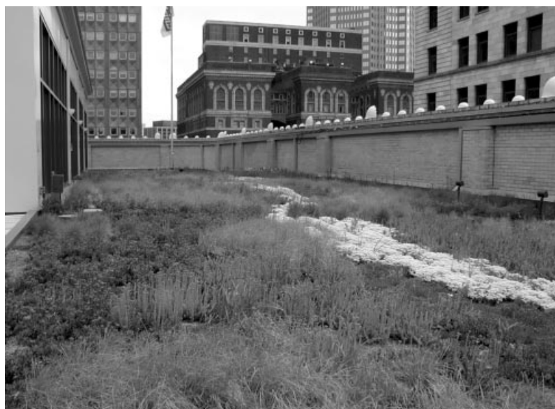
Heinz 57 Center, building restoration, Pittsburgh ROOFSCAPES, INC.
