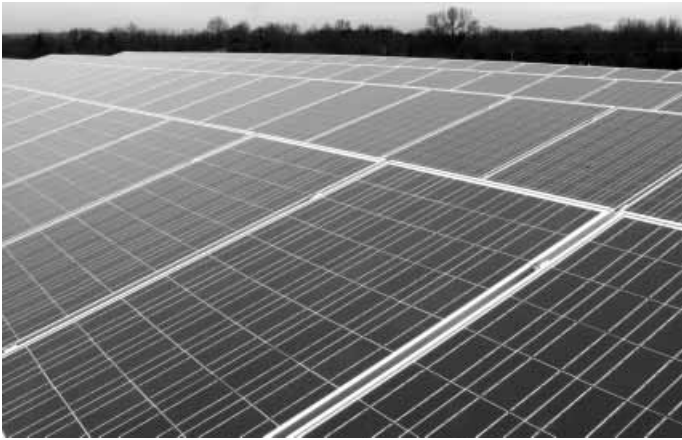
Large scale solar developers propose to cover thousands of acres of South Jersey farmland.
